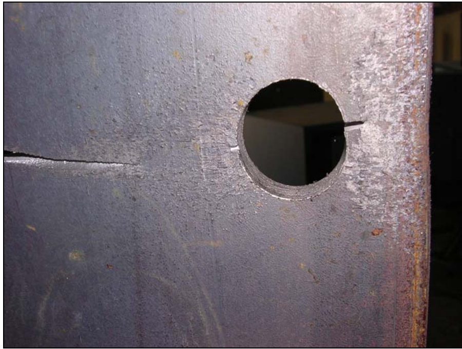
Figure 5.11: Profile Close-Up of Fatigue Crack
